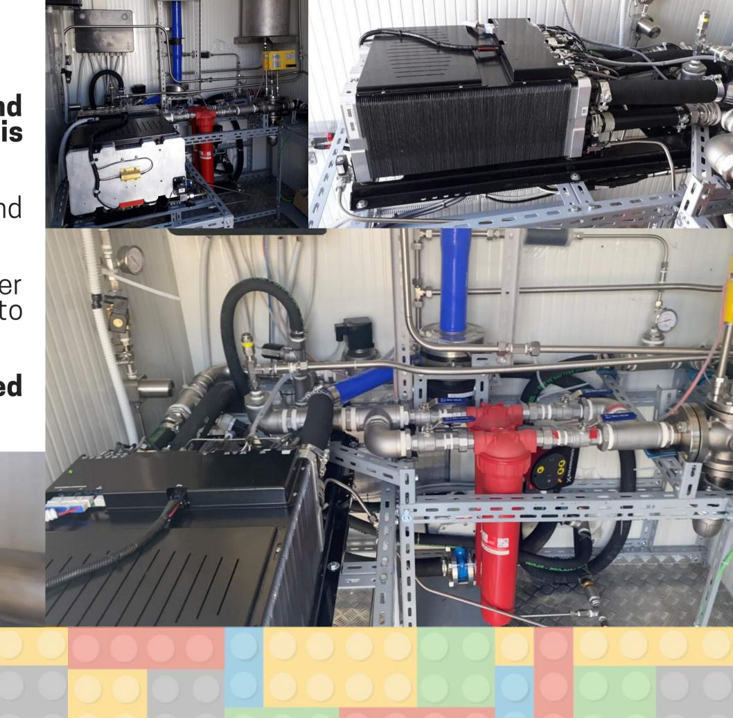
**CONVERT module:** Electricity generted from renewables is converted in Hydrogen (chemical energy) and sent to the STORE module.
